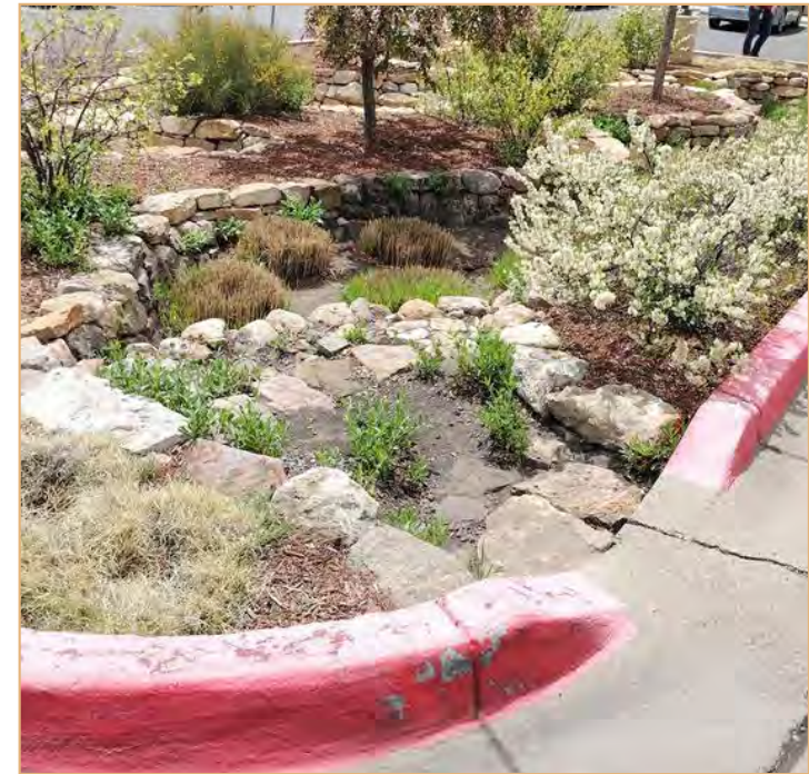
Figure 88: Center Median Runoff Capture and Infiltration
