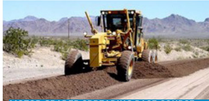
MOTOR GRADER SPREADING BASE COURSE
