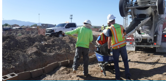
FIELD SAMPLING FOR CONCRETE TESTING
