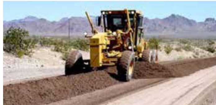
MOTOR GRADER SPREADING BASE COURSE
