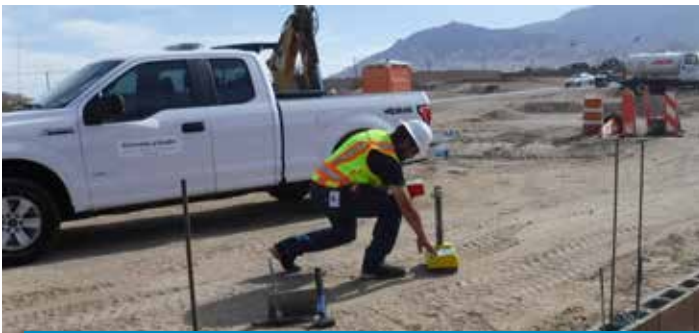
DENSITY AND MOISTURE TESTING FOR COMPACTION
