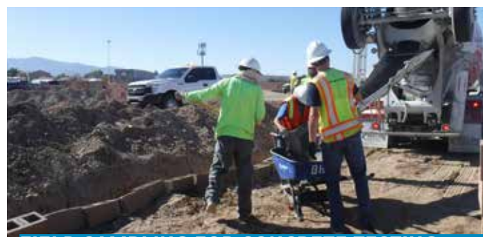
FIELD SAMPLING FOR CONCRETE TESTING
